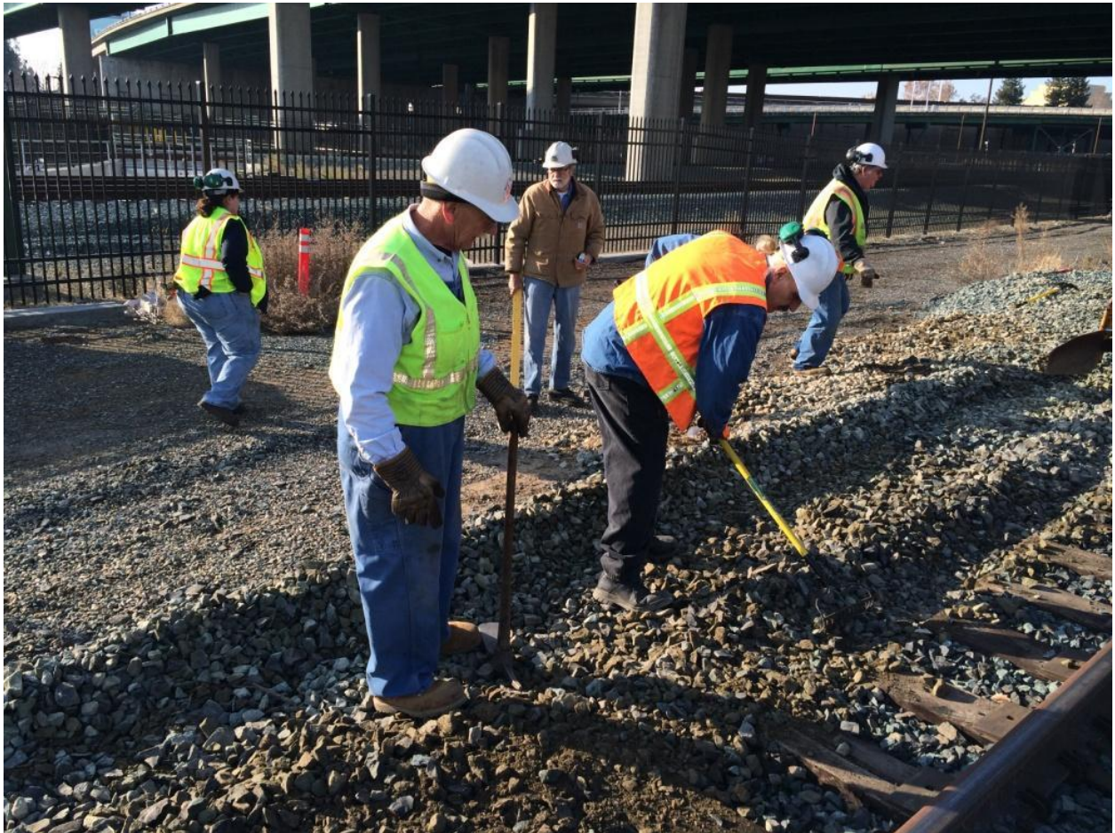
Clem and Fred were tireless in their efforts to shovel rock around the switch
