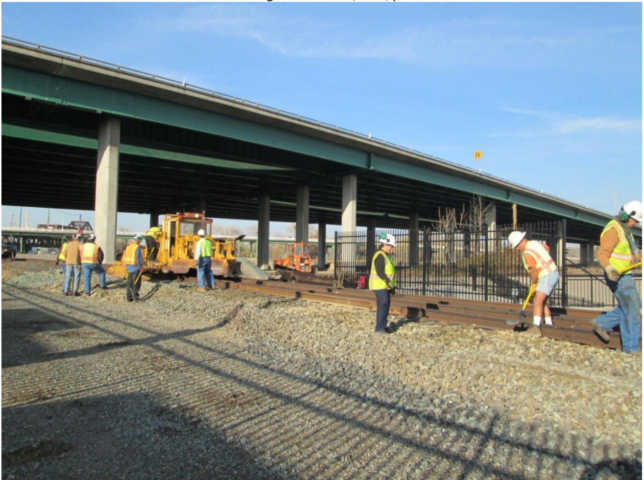
Shifting rock by hand is a team effort – especially while trying to make emergency repairs to the regulator...
