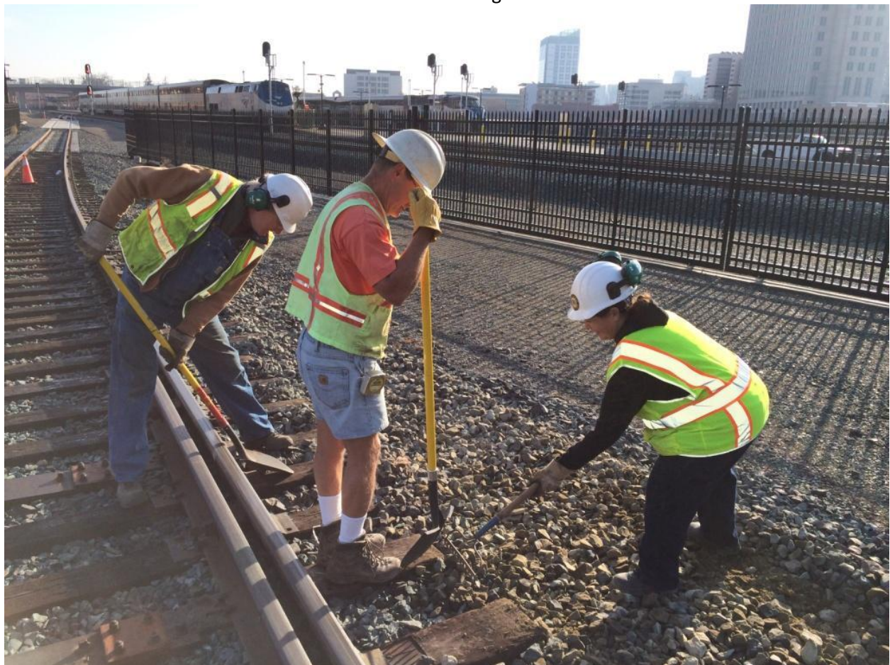
Steve N., Steve M., and Pam cut away at the slope by hand at the switch
