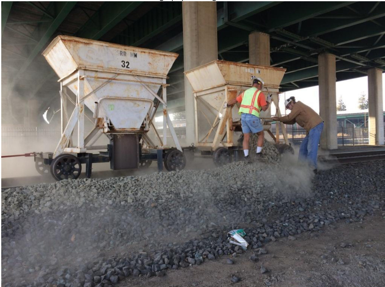
Steve M. and Alan "ballast" the track
